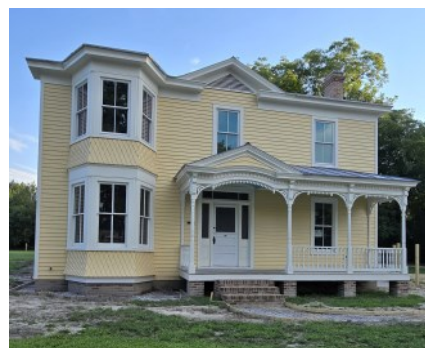
Restored Farinholt House
